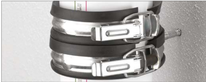
Fig. 12-1 Patented structure-borne sound-dampening support bracket
