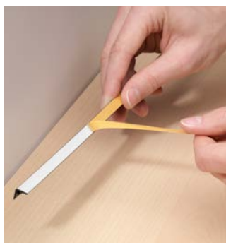
2. Remove adhesive tape
