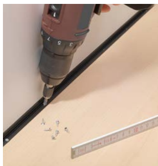
4. Screw into place (chip board screw countersunk 2.5x10 )
